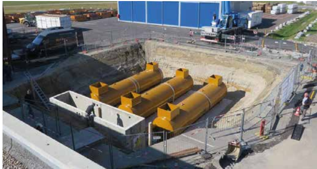
Three new underground wastewater collection tanks with 30m 3 each capacity
