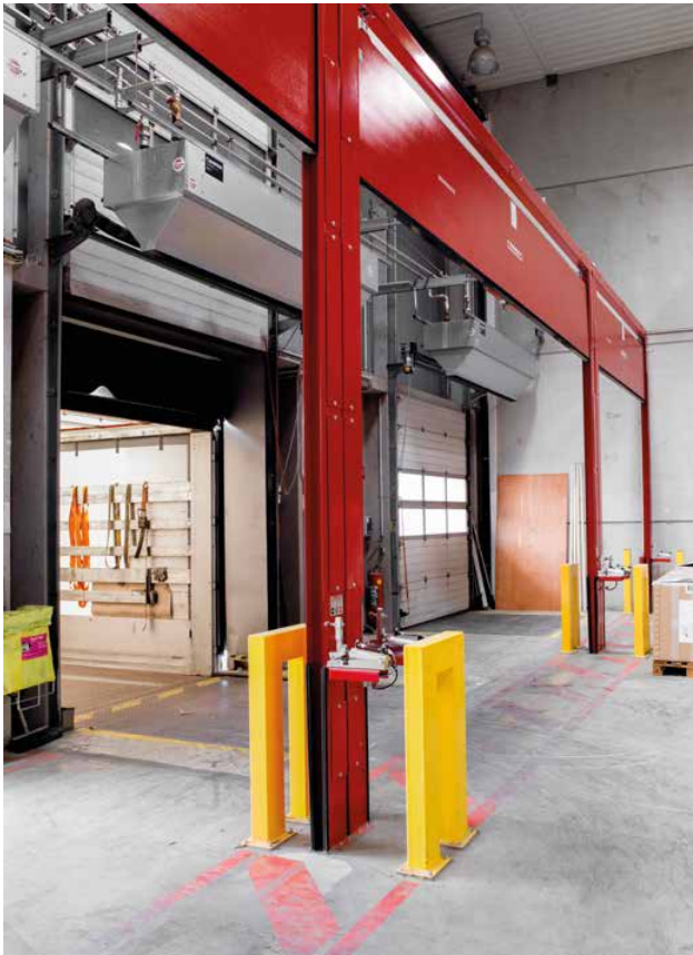
Firewater retention barriers at all exits
