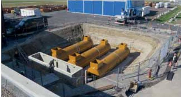
Three new underground wastewater collection tanks with 30m<sup>3</sup> each capacity
