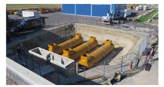
Three new underground wastewater collection tanks with 30m³ each capacity
