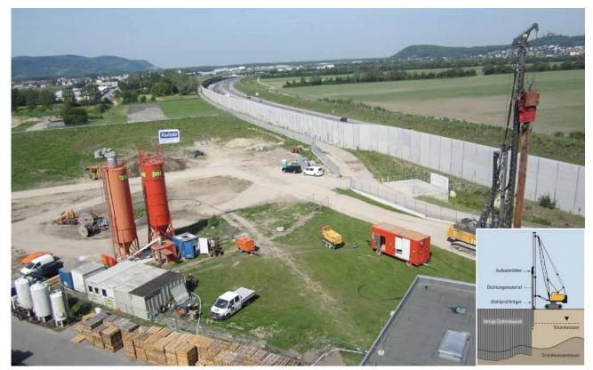
Rammer with suspension silos
